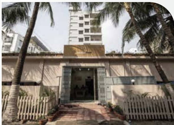
Alok Nibash 1 Building.
