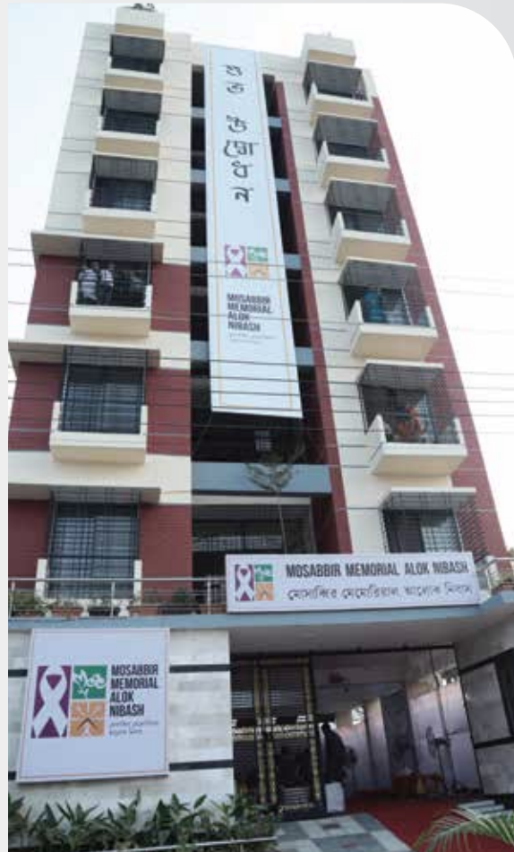
Alok Nibash 2 Building.
